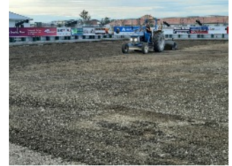
The soil has gone, the base course is complete and levelling and rolling continues.
