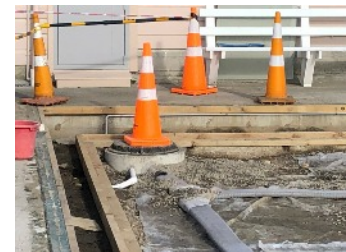
The soil has gone, the base course is complete and levelling and rolling continues.
